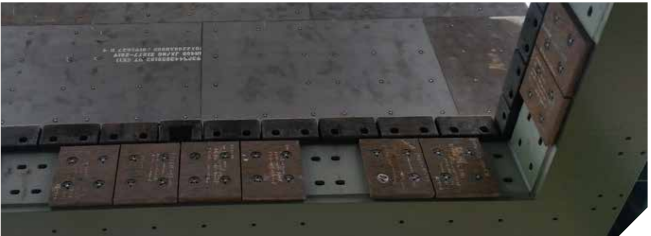
Liners being installed using the Taper-T attachment system.
