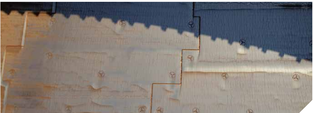
Taper-T attachments in service showing minimal preferential wear.
